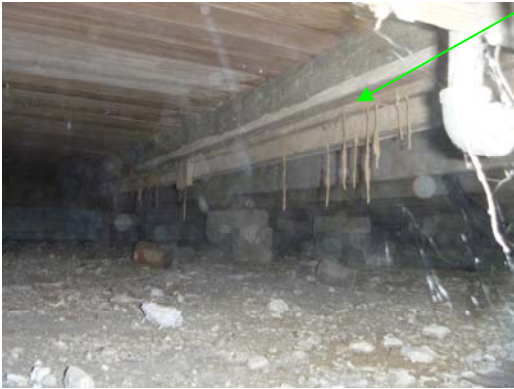
Termite damage to structural beam
