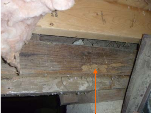
Termite damage to structural beam
