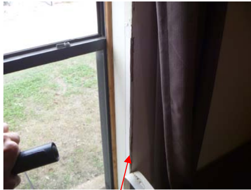
Window sill trim and sheetrock
