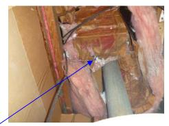
X Fire blocking (fire-rated sheetrock, plywood, etc) missing at ceiling for HVAC/Water Heater Closet in garage. This ceiling helps contain flames from spreading into the attic.
